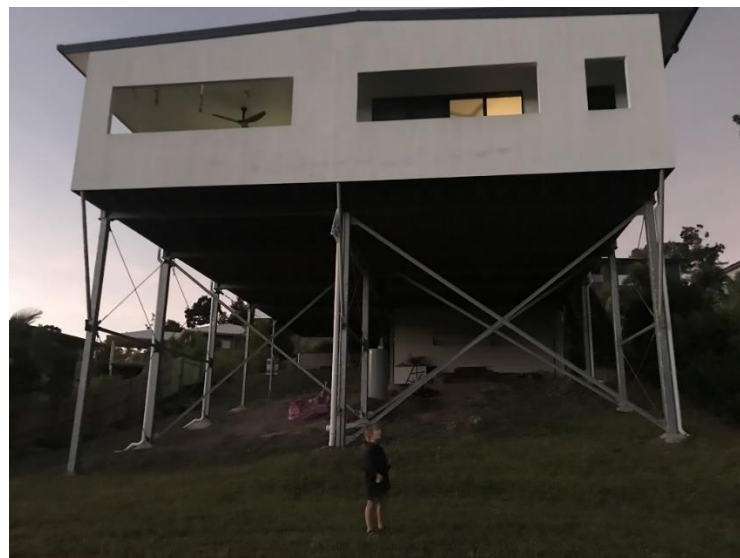
Fig. 7. The finished design of the Airlie house
