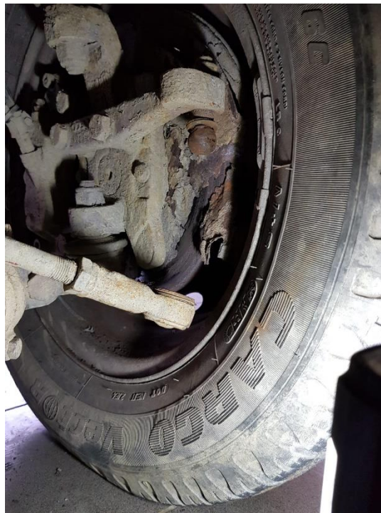
Fig. 2. An example of complete destruction of a ball joint
