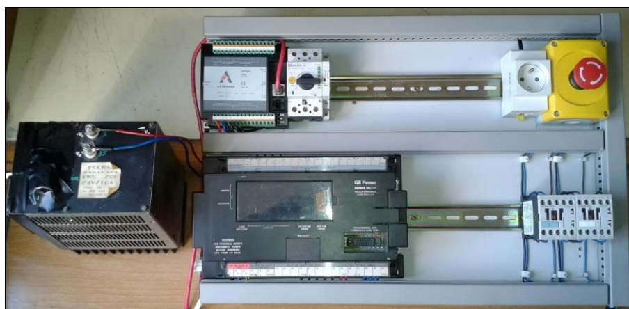
Fig. 7. View of the control system
