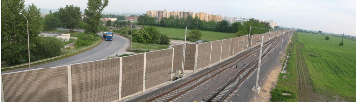
Fig. 15. View of the noise barrier
