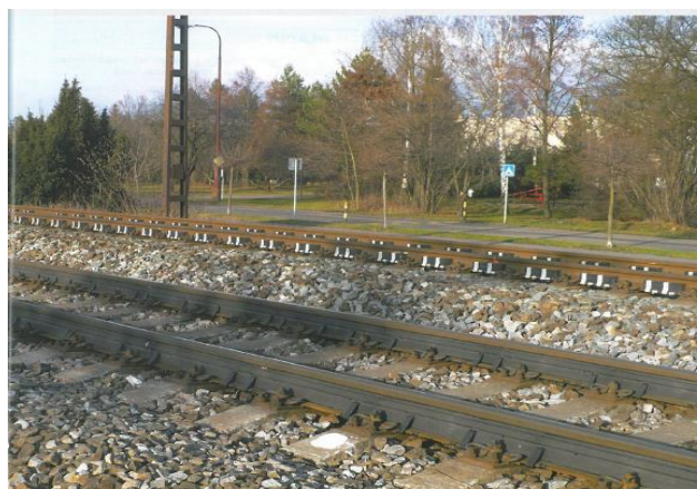
Fig. 14. Rail absorber Vossloh and Corus [11]
