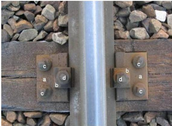
Fig. 1. Screw fastening of the K type, a-the rib plate, b-trap hook, c-fastening screw of the rib plate, d-bolt with nut [3]
