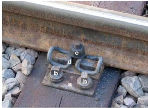
Fig. 2. Spring spikes or elastic rail system SKL 12, a-ribbed plate, b-screws that secure the backing plate rib, c-hex nut, d-elastic clip SKL 12 [3]
