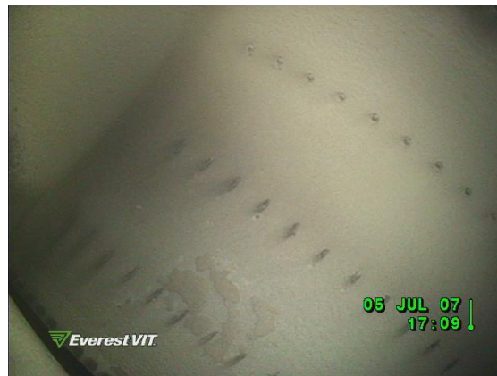
Fig. 8. Coating missing from the high-pressure turbine blade's concave side due to flaking
