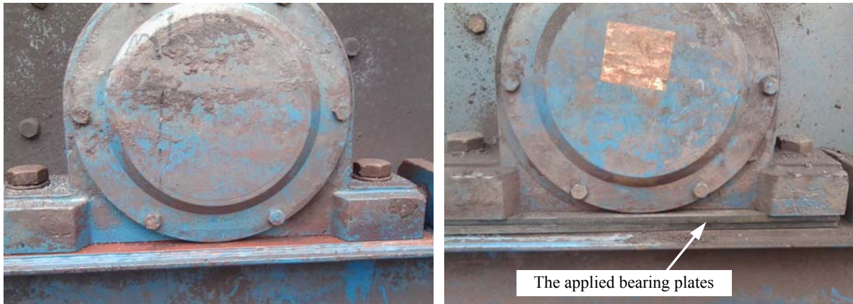
Fig. 5. Elimination of the angular deviation in the vertical plane
